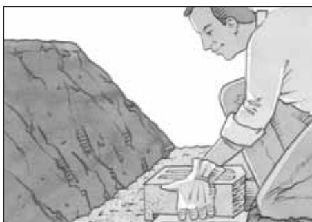
CONSTRUCTION OF THE NEXT COURSE
