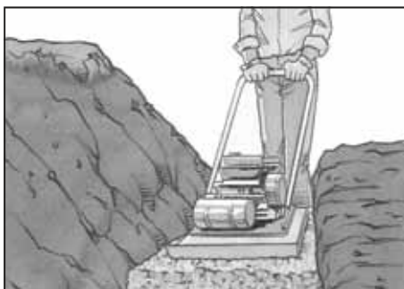
LEVELLING PAD (FOOTING) COMPACTION
